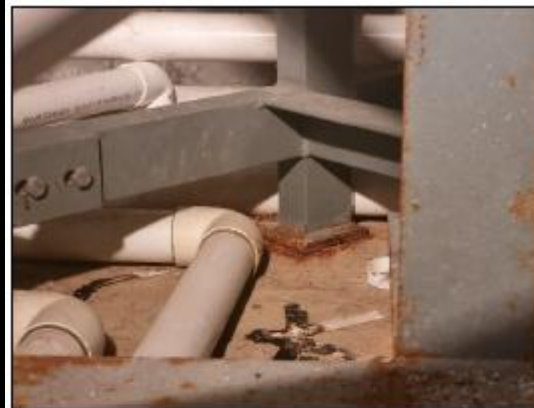
Photo 2 – Corrosion to steel baseplate of the Spa support frame
